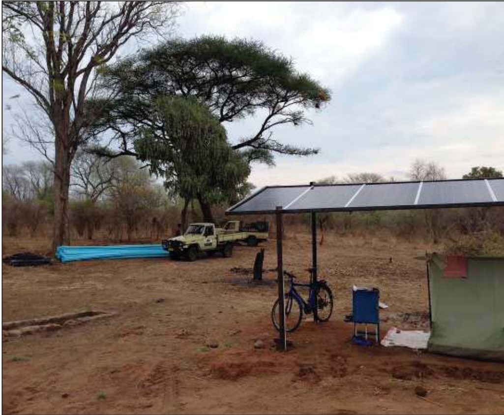
*** 3200m of piping and solar pump installation Dande East, October 2018***
